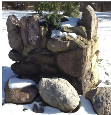
Unrestored Stone Pier, 2013.
