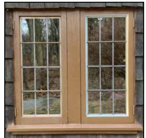
Restored windows on the North Cottage.
